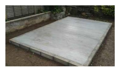
The concrete base is 350-400mm deep. We use type 1 hardcore on the base then sand which is compacted down before we fit a damp proof membrane before pouring the concrete to the height 70mm below finished floor level. We lay floor joist and Kingspan boards then fit the flooring.
